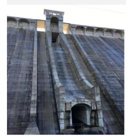
All dams have a spillway at the crest that act as a safety limit in case of maximum filling of the reservoir. Sometimes the maximum level needs to be variable and is normally controlled by opening or closing the spillway gates. However, the variable level is limited by the height of the gates.
